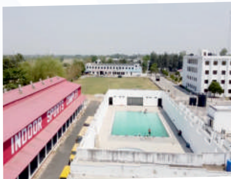
Indoor Stadium & Olympic Size Swimming Pool
